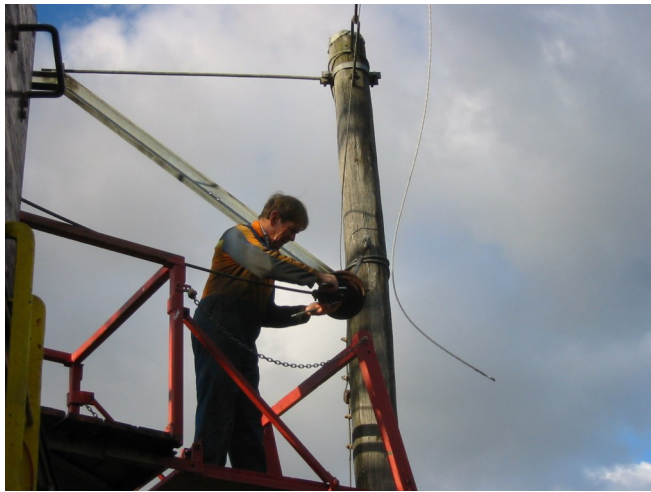
Above left: Joe in action installing a disk insulator on a pole during the Overhead line installation to Ferrymead station.
