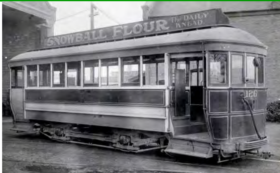
ABOVE: The first of a new generation. The first 'Standard' trailer, No. 126 at Falsgrave Street depot on its entry to service, c. 1917. Originally fitted with the same aluminium blinds as the 'Dreadnought' and 'Big Berthas' on its end platforms, these were later replaced by two-part doors. Withdrawn in 1954, No. 126 was sold for use as a holiday home on Banks Peninsula before being acquired by THS for preservation. Photo: Graham Stewart collection.
