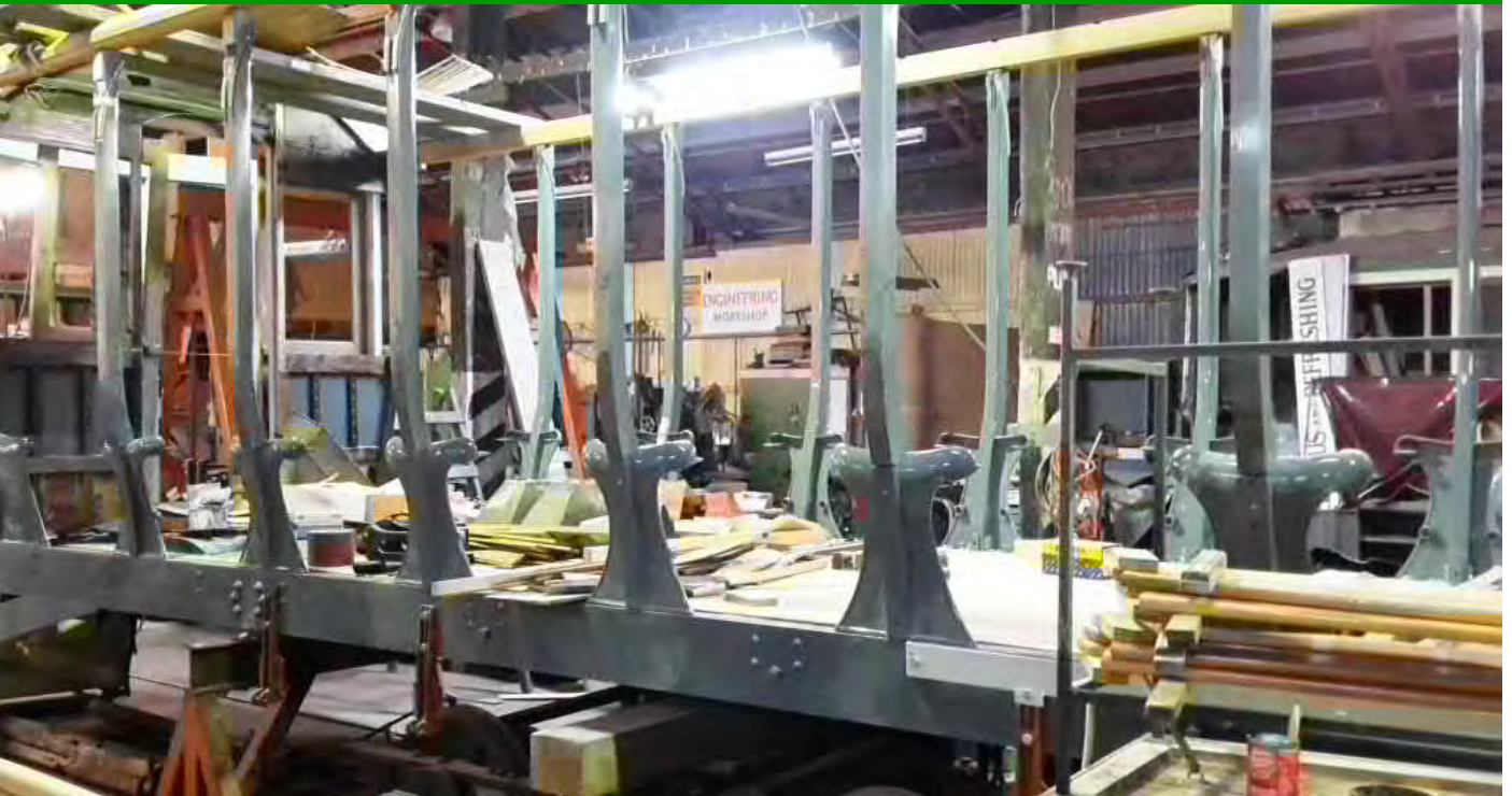
ABOVE: Earlier this month, Stephen Taylor and his team restoring CTB ‘Hills’ car 24 completed the installation of the roof pillars and seat bases in the convertible section. Photographed on 12 September 2016, shortly after the last parts had been finally installed. Photo: Stephen Taylor.
