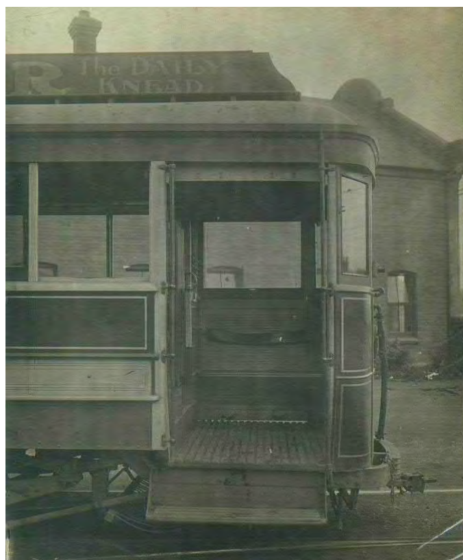
ABOVE: A closer view of the aluminium sliding panel and window arrangement on the end platform of No. 126. Less than reliable in service, they were soon taken out and replaced with normal doors.
