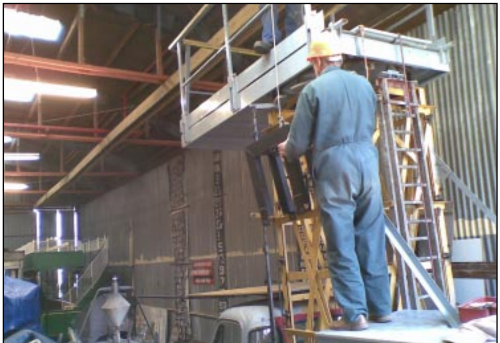
Middle: one of the new brackets in position. The section of the cross beam under the bracket has yet to be removed.
