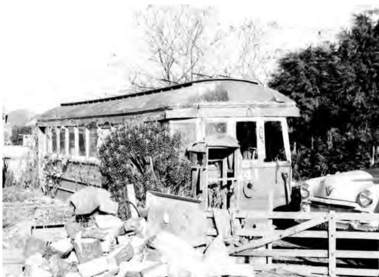
ABOVE: The wreck. The remains of 'Standard' 141 at Tancred Street, Ashburton, showing the accident-damaged No. 1 end.
