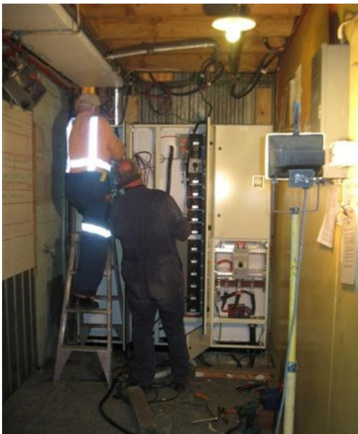
Brian Lester and Brian Fairbrass feeding cables into the distribution board. Photo: Murray Sanders.
