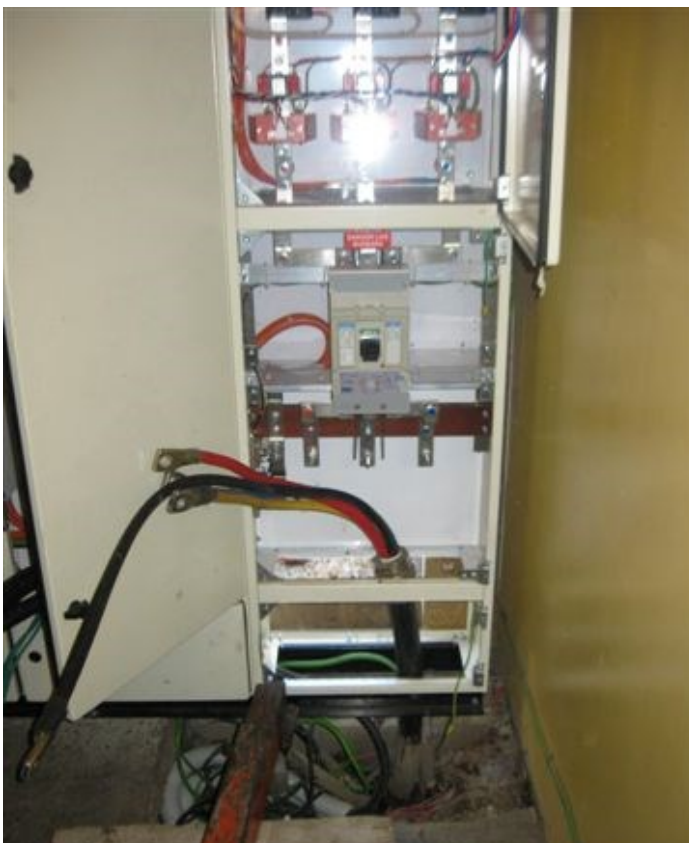
Aluminium mains conductors ready to be terminated. Photo: Murray Sanders.
