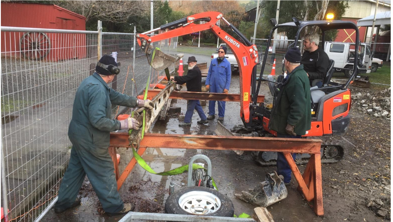
ABOVE: Jonathan Day and team hard at work on the Hall of Wheels siding points on Saturday 15 June; while the blade, mate and frog are out of the ground, the team will clean them up and weld up some cracks as noted previously. PHOTO: Dave Hinman.
