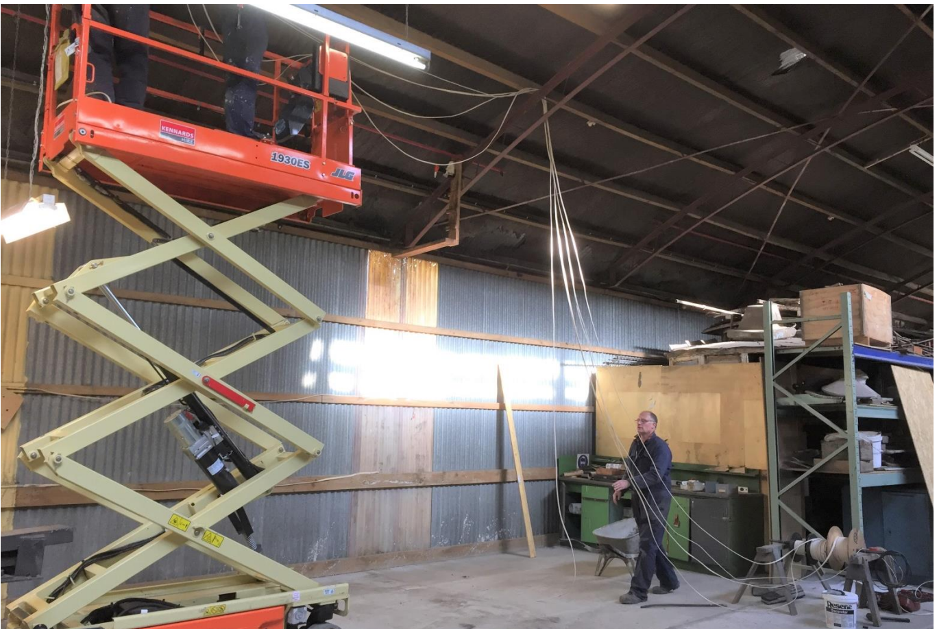
BELOW: Graeme Richardson assisting Murray Sanders and Wayne Fisher (partly visible) with the installation of the new cabling being installed to power the new equipment. We hope to publish a description of what new equipment has been installed, and what prerequisites are required for using it (if any), in a future issue. PHOTO: Dave Hinman
