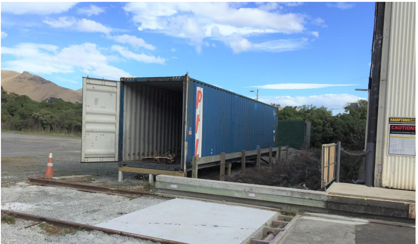
BELOW: Further down the traverser pit, a 40ft container has been installed for 'Yank' 12 to live in between bouts of periodic restoration. Yet to be constructed is the bridge that will allow N o 12 to be rolled off the traverser and into the container, though this likely won't be too far away. PHOTO: Dave Hinman.
