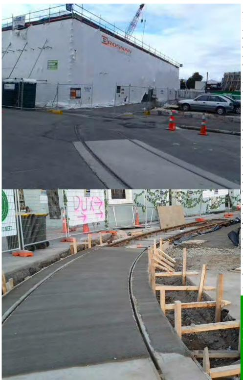
**RIGHT** and **LOWER RIGHT**: Before the start of work at Lichfield Street and Poplar Lane, the start of the new tramway curve as well as the track down Poplar Lane had already been installed as part of the work pre-February 2011. The 6.3-magnitude earthquake of 22 February 2011 subsequently halted any plans to construct the 'missing' curve between these two sections of track.
