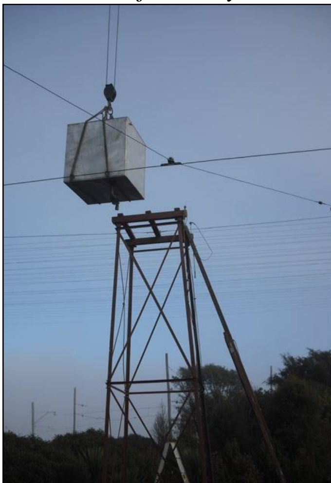
On a foggy Saturday, the new tank stand to supply water for Kitty's thirsty boiler was stood up. When commissioned, it will enable Kitty to be revictualled at the platform instead of having to be withdrawn to the side of the tram barn..
